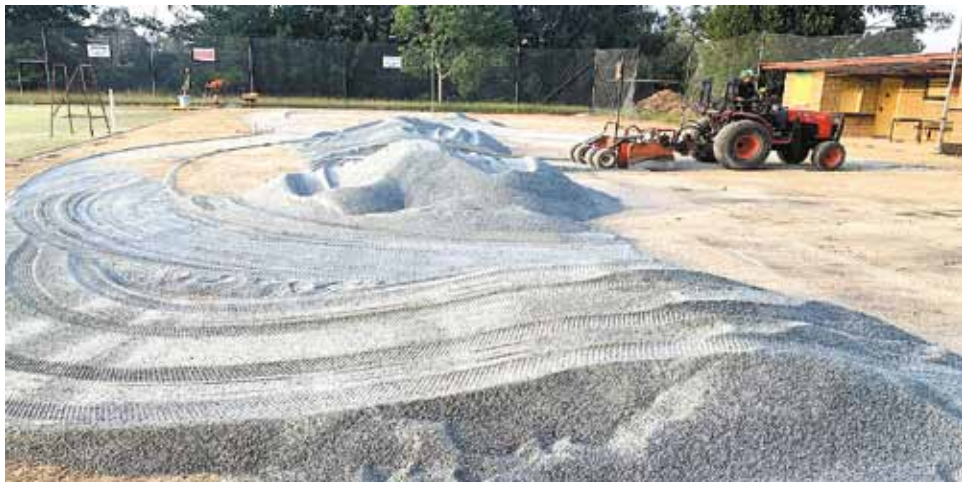
Works in progress, replacing Court One
