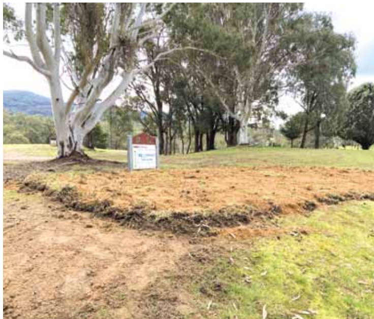
The ladies 2 nd tee under repair
