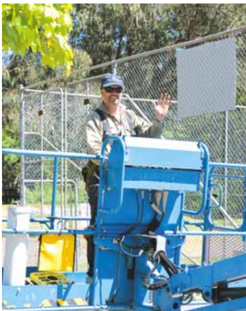
Rob Gollan of EDC Electrical installing the new LED lights
