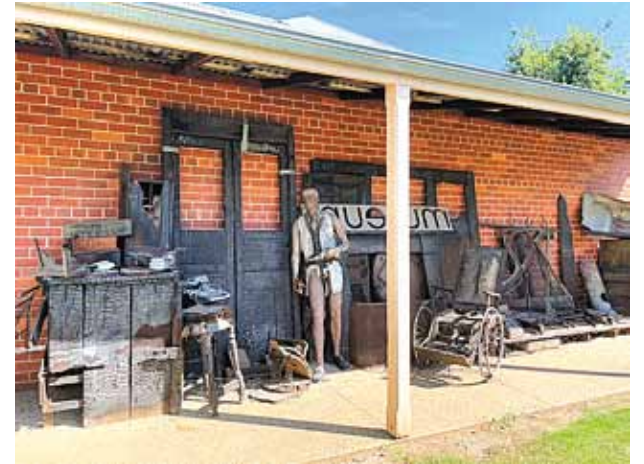
Items damaged by the fire in 2006, now ready for a new lease of life
