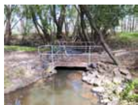
The Jackson/Klose Culvert on Back Creek
