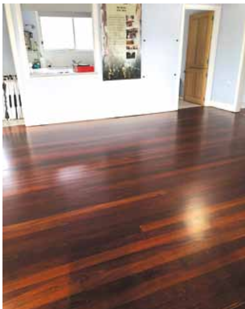
The restored timber flooring at Bruarong Community Centre
