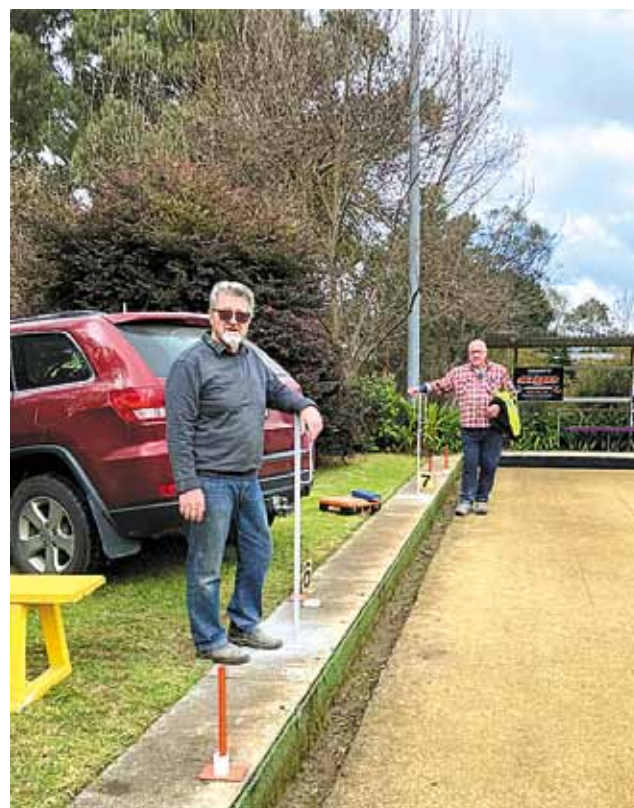
Mike Tobin and Reon Garvey complete the safety rails
