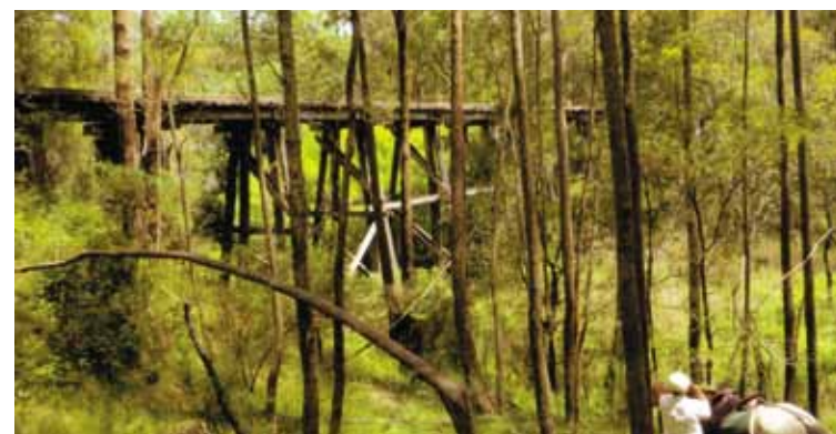
Boggy Creek trestle bridge
