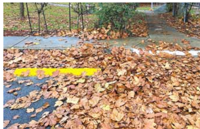
Repainted wheel stop kerbing - thanks to Indigo Shire Council
