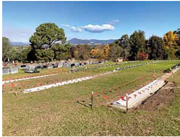
Extending the headstone beams
